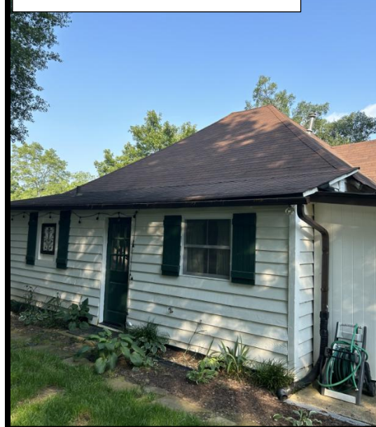
Existing Conditions (Rear)
