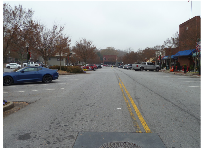
Photo 5: Looking north in downtown section of South Peachtree Street from Holcomb Bridge Rd.
