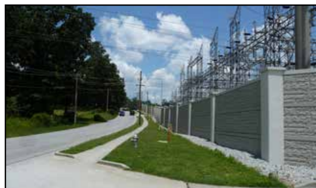
Photo 6 - The existing sidewalk on N. Norcross Tucker Road can be replaced with a multi-use trail to access the neighborhoods along that street.
