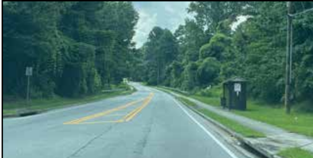
Photo 4 - Southbound view on Mitchell Road, just north of the Beaver Ruin Creek culvert.
