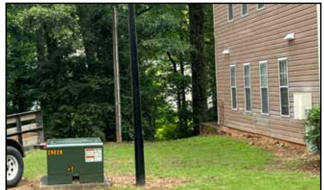
Photo 9 - Due to steep grades, it is impractical to install a trail to connect the back of Brook Hollow Apartments to Western Hills Drive (Area K)
