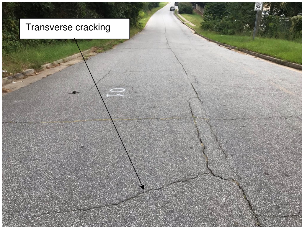
Photo 2. View of typical pavement condition at C-1
