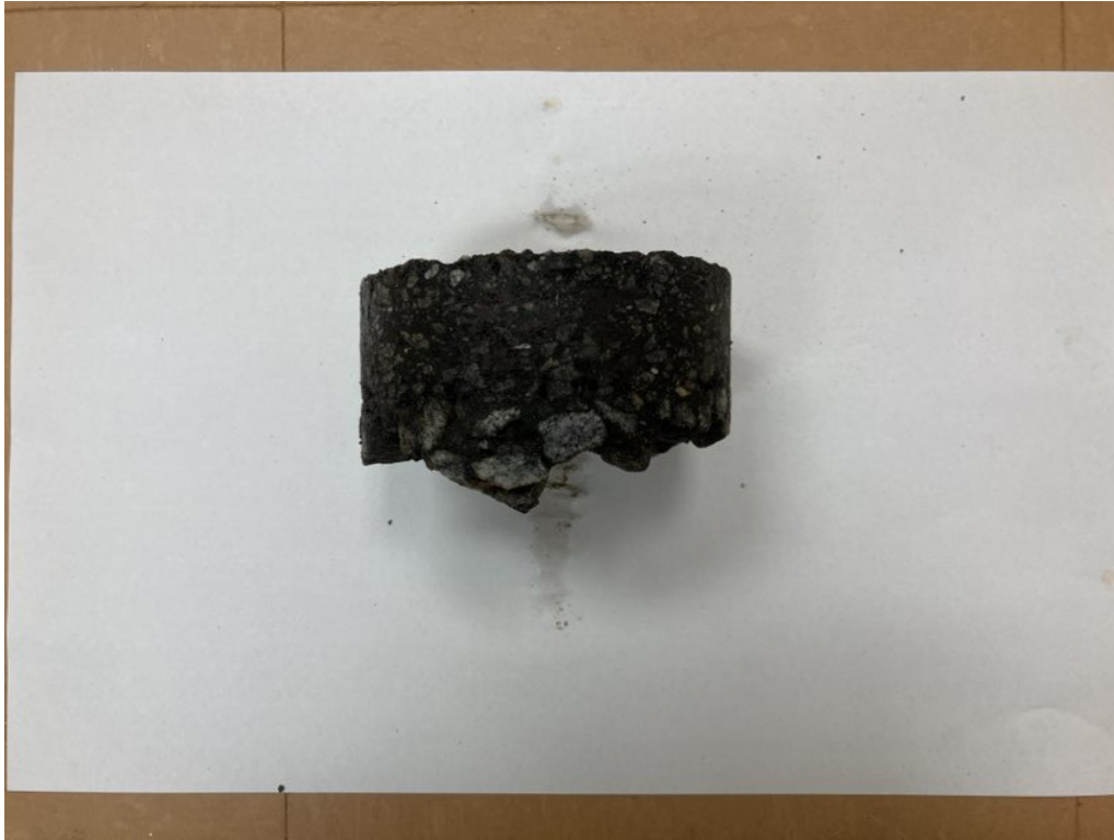
Photo 5. Core C-5. Asphalt Thickness = 2 inches
