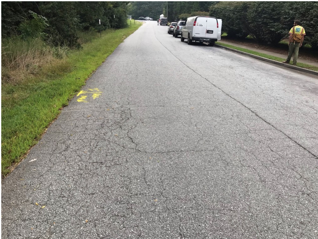
Photo 6. View of typical pavement condition at C-3
