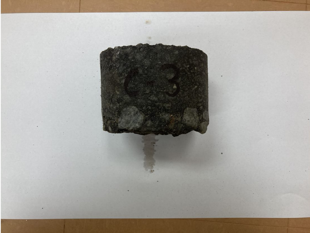
Photo 3. Core C-3. Asphalt Thickness = 3 inches
