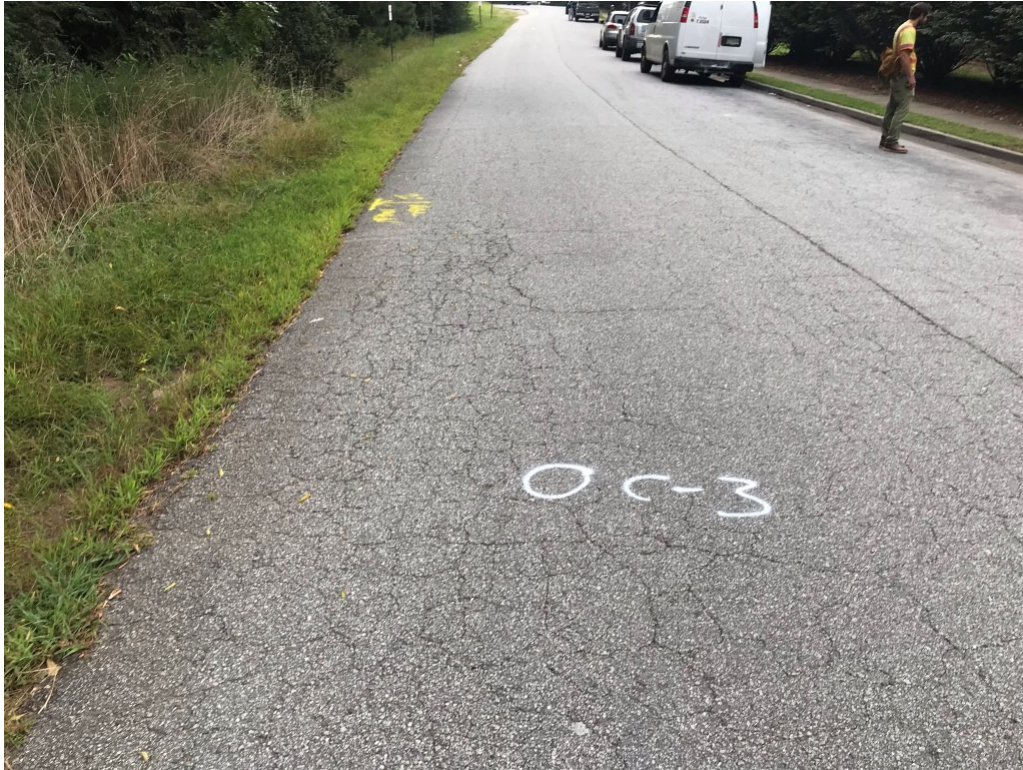
Photo 5. View of Core Location C-3 (Northwest bound lane)
