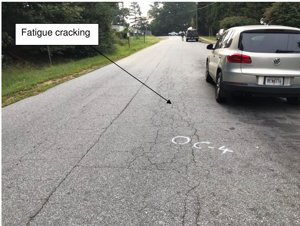
Photo 8. View of typical pavement condition at C-4
