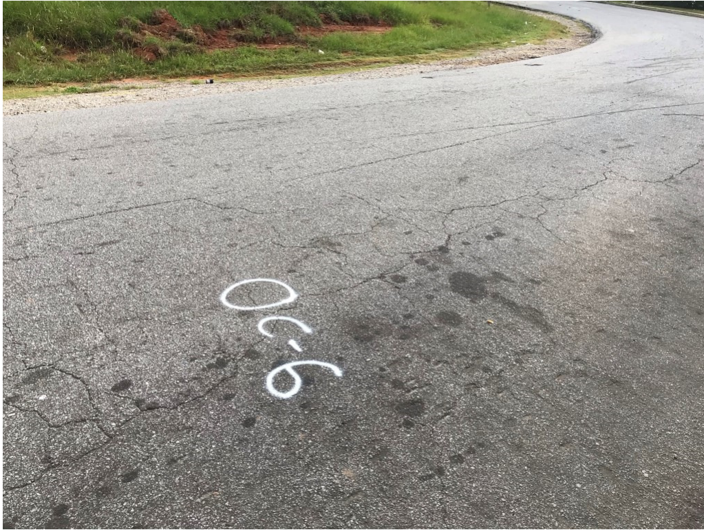
Photo 11. View of Core Location C-6 – (Southeast bound lane)
