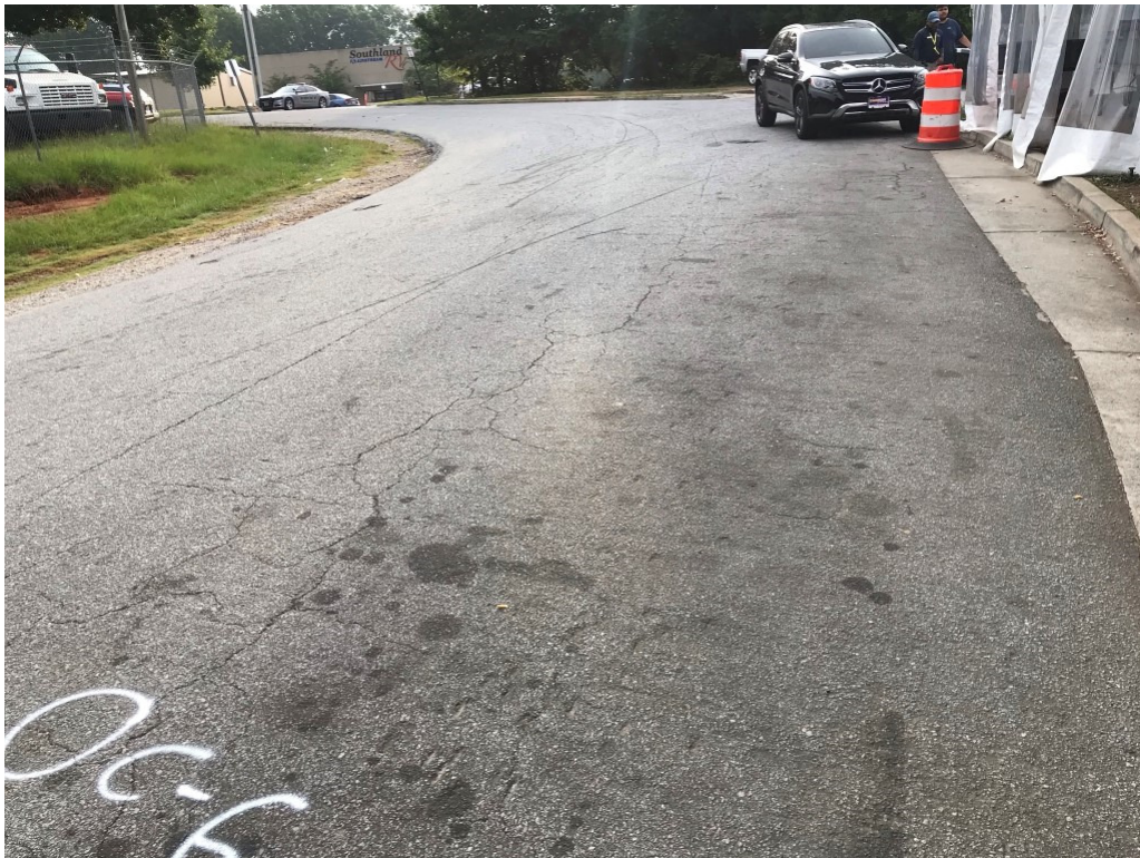
Photo 12. View of typical pavement condition at C-6
