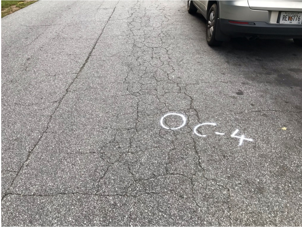
Photo 7. View of Core Location C-4 (Southeast bound lane)
