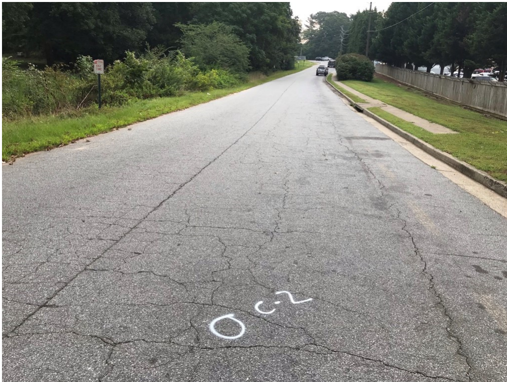
Photo 4. View of typical pavement condition at C-2
