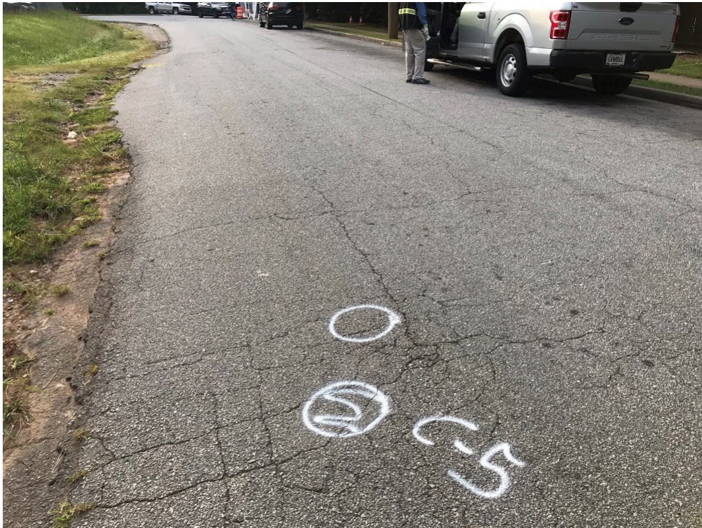
Photo 10. View of typical pavement condition at C-5
