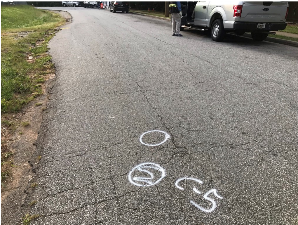
Photo 10. View of typical pavement condition at C-5
