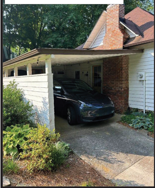
Existing Conditions (Left)
