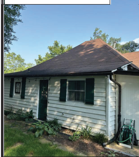
Existing Conditions (Rear)
