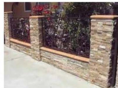
Masonry and wrought iron
