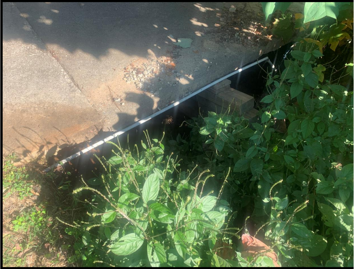
Attachment: Photos 5946 Hammond Drive (24-7176 : Storm Water Pipe Repair and
