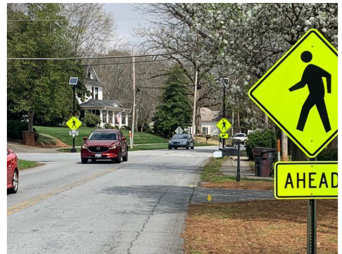
Photo 12: Existing Pedestrian Crossing with Warning System at Sunset Drive
