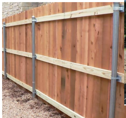
Steel Posts with Wood Pickets Using Conversion Brackets
