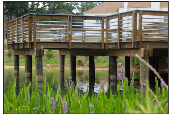
Boardwalk & Outdoor Classroom
