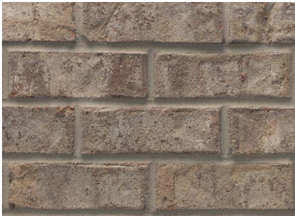
Mountain Brooke Brick with Coosa Light Mortar
