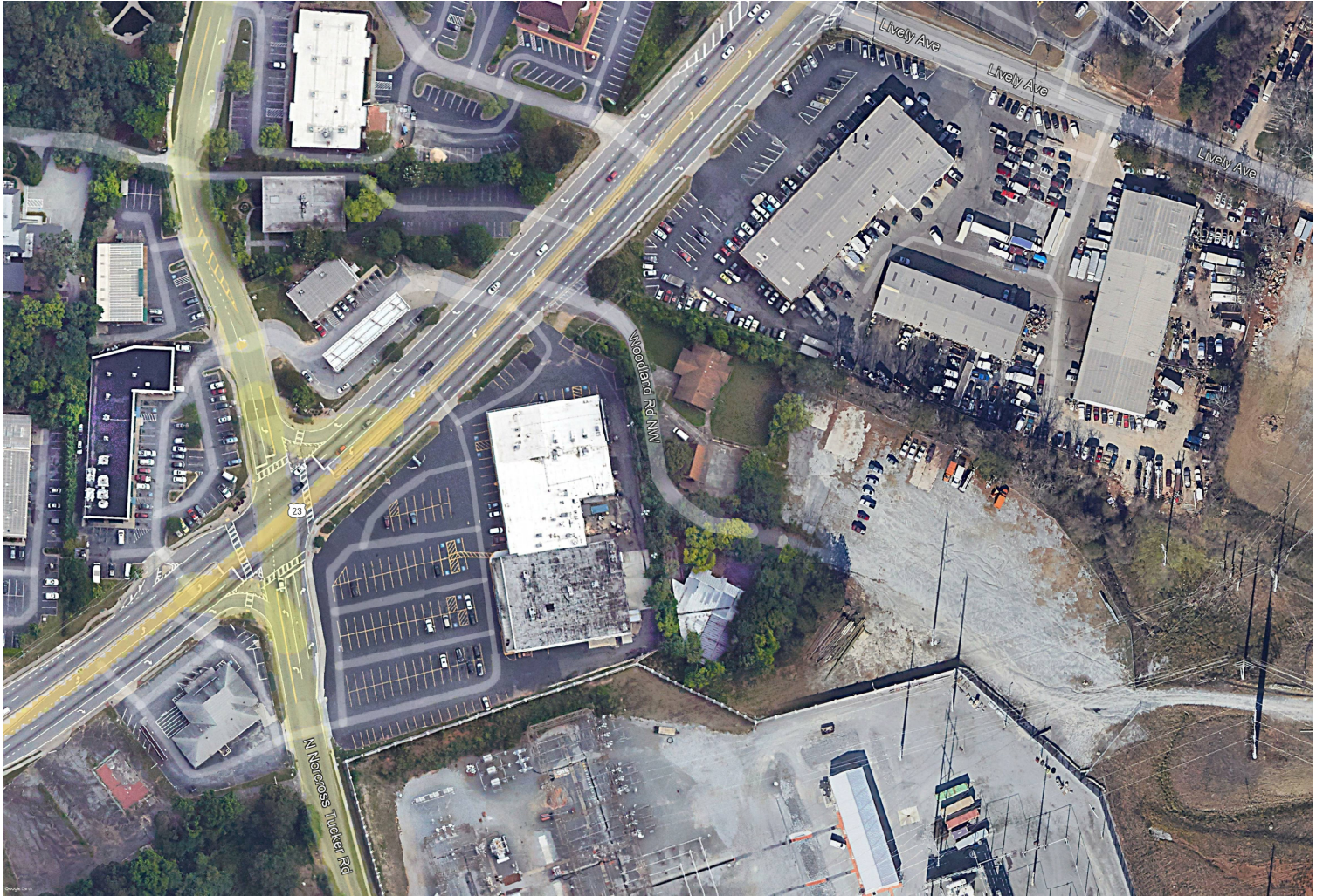
Attachment: ITB PWUP 24-03 - SPLOST (24-6949 : SPLOST Transportation Resurfacing)
