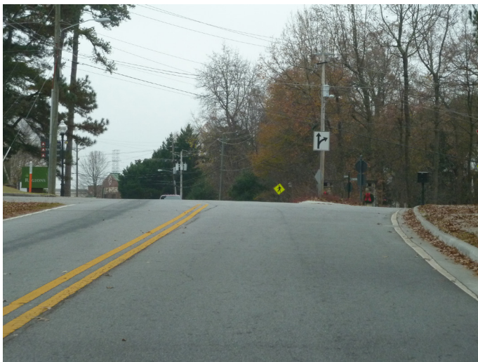
Photo 6: Looking west at split between South Peachtree St (RT) and Norcross Tucker (LT)
