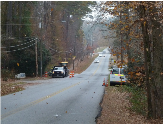
Photo 2: Looking east on Holcomb Bridge west of Christ Church Episcopal, showing typical 2-lane section
