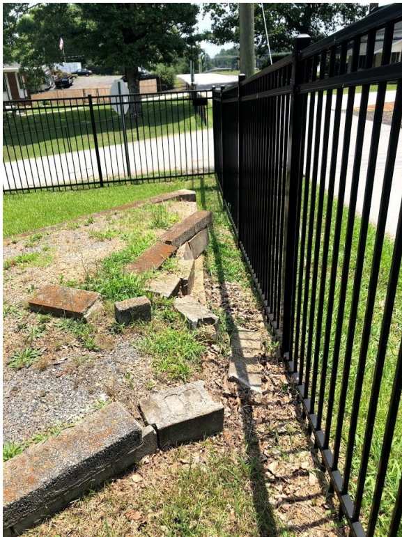
Action: Rebuild or ideally regrade both of these areas, burying coping/foundations where necessary
