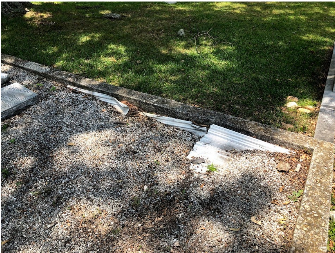
Action: Install additional pea gravel to cover aluminum
