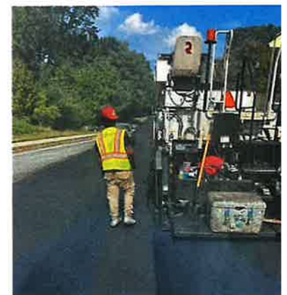
Paver on James Burgess rd.
