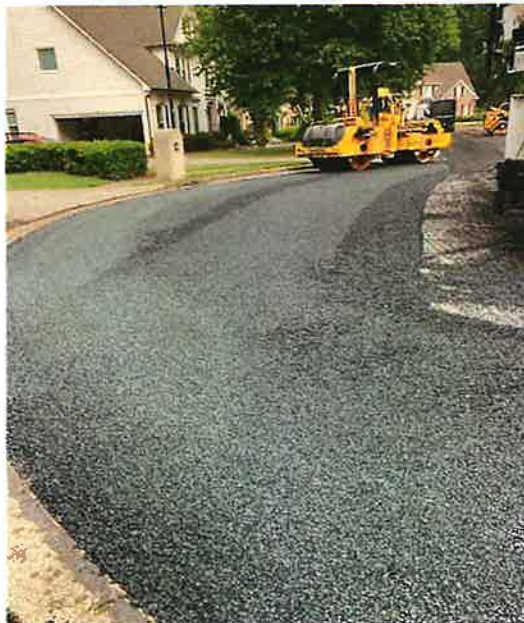
A roller underway on Barrick Lane Northwest
