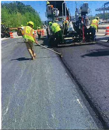
Asphalt Resurfacing April 2023
