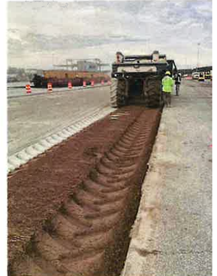
FDR work, also March 2023
