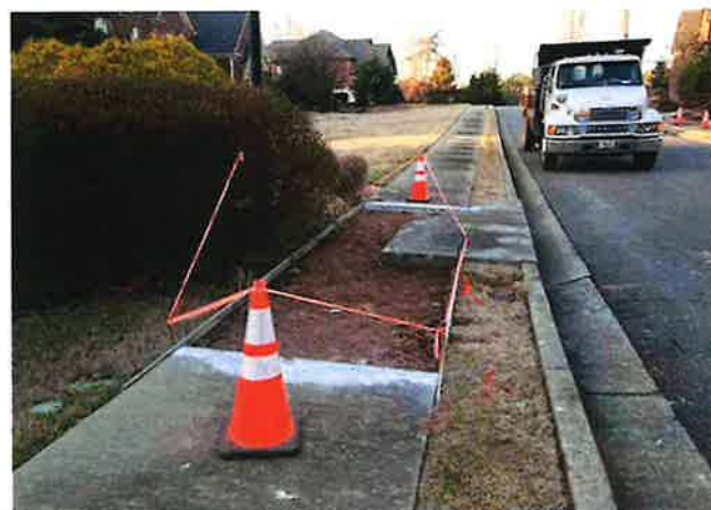
Concrete Replacement on Bethany Bend Road Milton, GA November 2022
