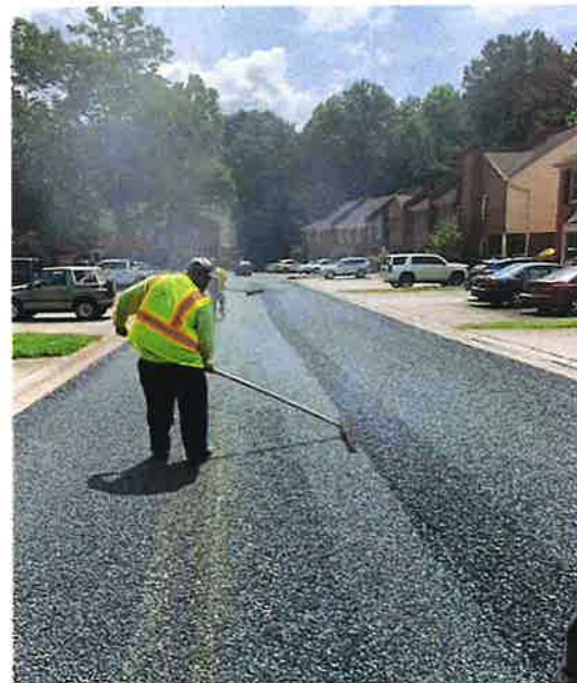
Paving Operations on Corner Oak Drive
