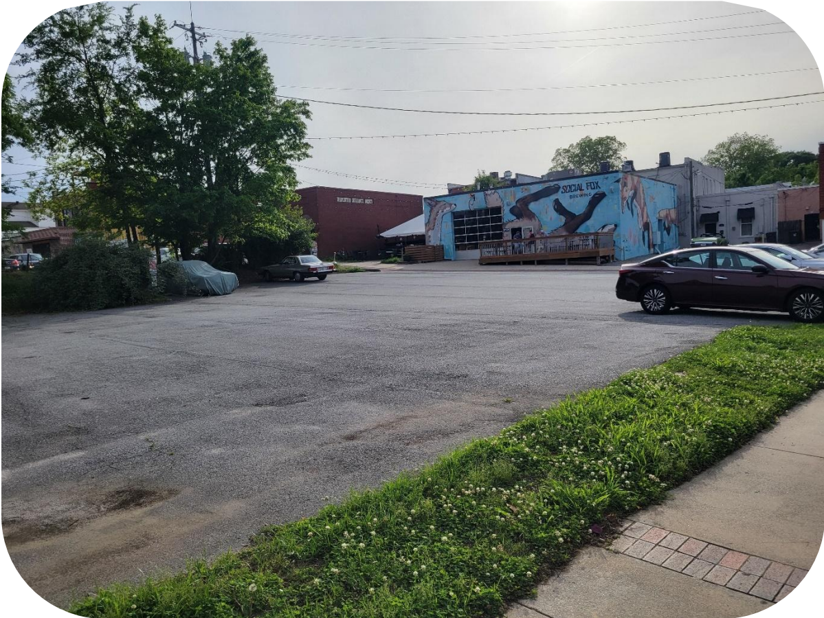
Figure 5. Limited Access Facility Resulting in Low Occupancy
