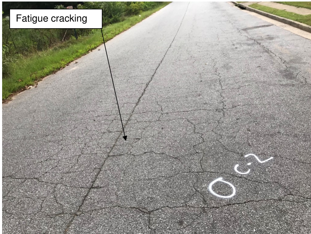
Photo 3. View of Core Location C-2 (Southeast bound lane)
