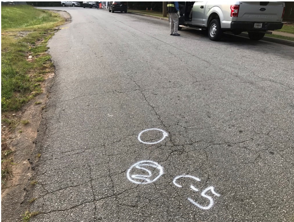
Photo 10. View of typical pavement condition at C-5
