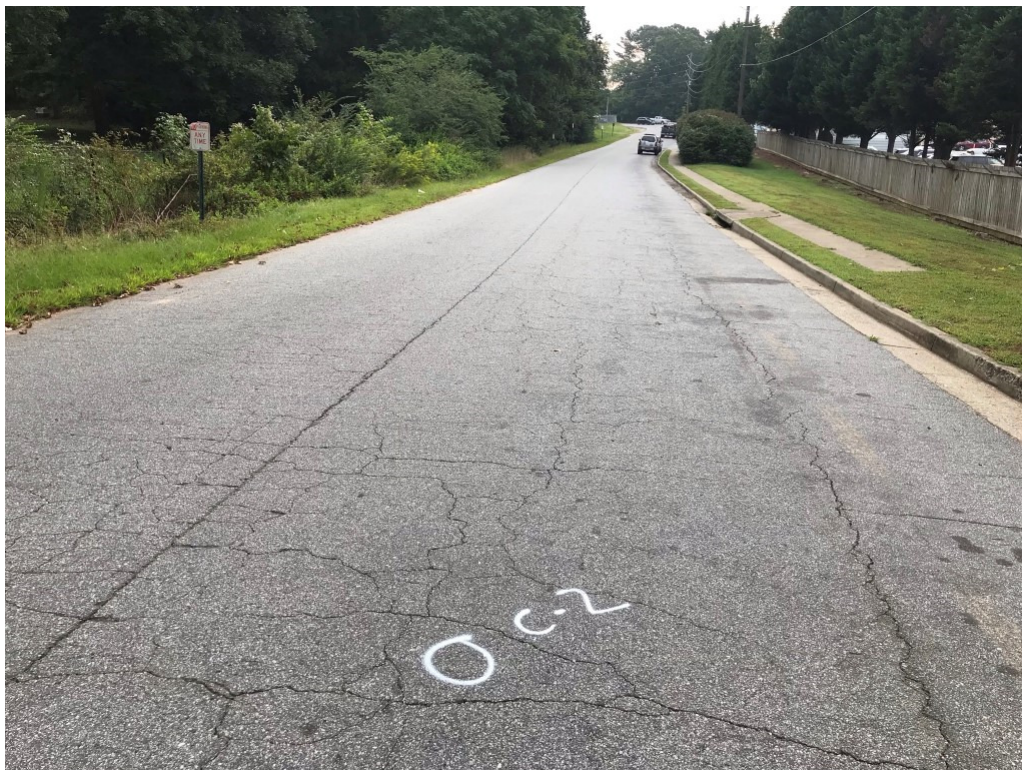
Photo 4. View of typical pavement condition at C-2
