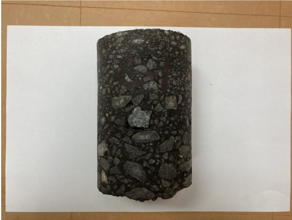
Photo 1. Core C-1. Asphalt Thickness = 7 inches
