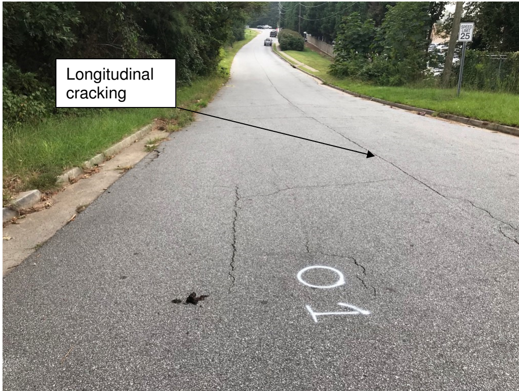
Photo 1. View of Core Location C-1 (Northwest bound lane)
