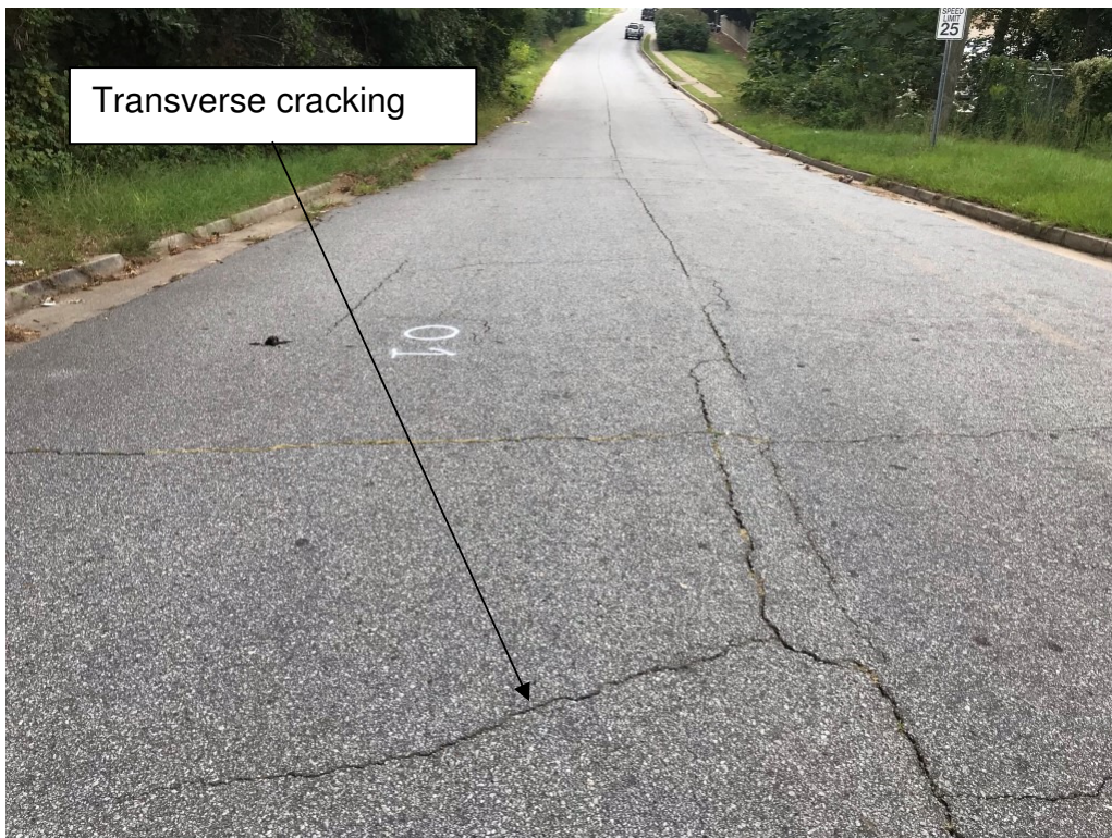
Photo 2. View of typical pavement condition at C-1
