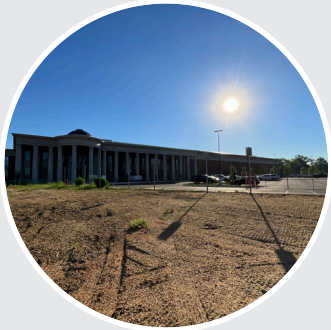
ENHANCED COMMISSIONING US Geological Survey's Hydrologic Instrumentation Laboratory, Tuscaloosa, AL
