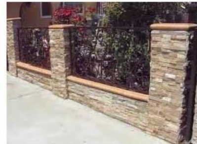
Masonry and wrought iron
