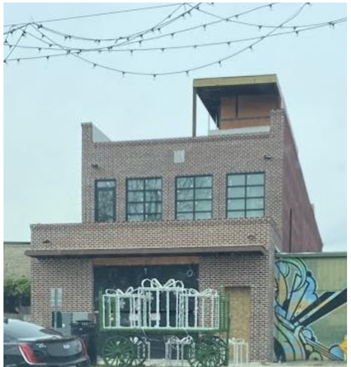
Existing Conditions – Photo Taken by Staff
