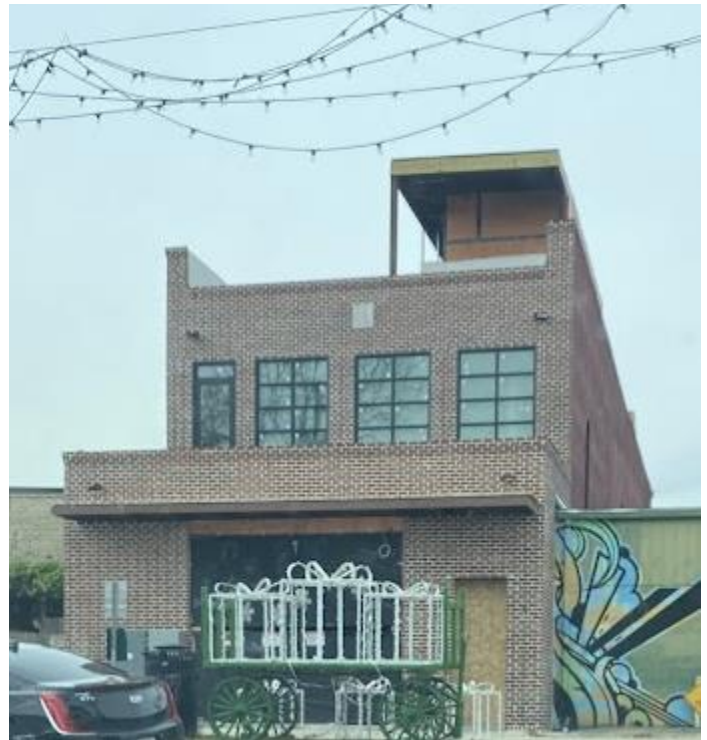
Existing Conditions – Photo Taken by Staff
