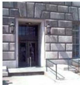
Entrance made accessible by adding inconspicuous ramp.
