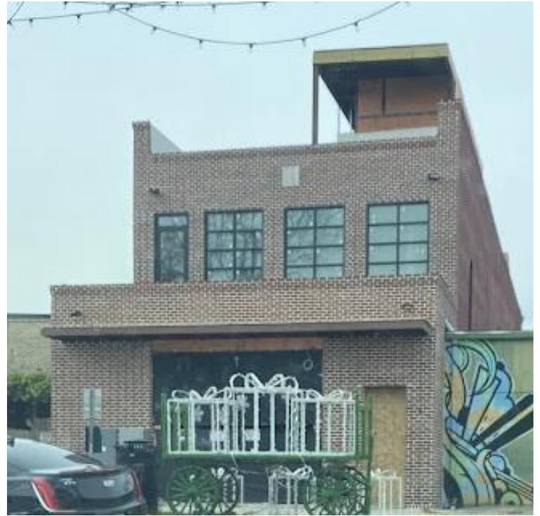
Existing Conditions – Photo Taken By Staff
