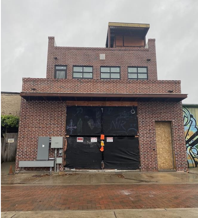
Existing Conditions – Photo Taken By Staff
