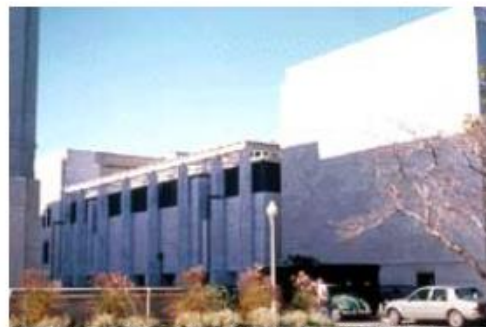
Contemporary addition (left) to historic library appropriately placed on secondary side elevation.
