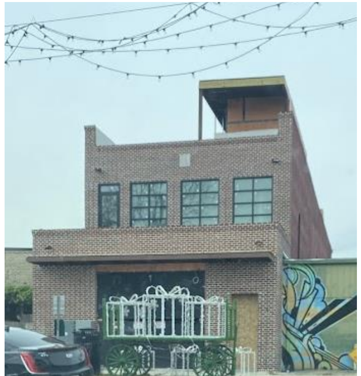
Existing Conditions – Photo Taken by Staff
