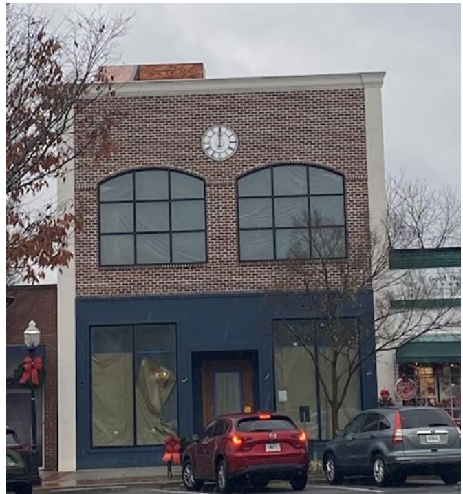
Existing Conditions – Photo Taken By Staff
