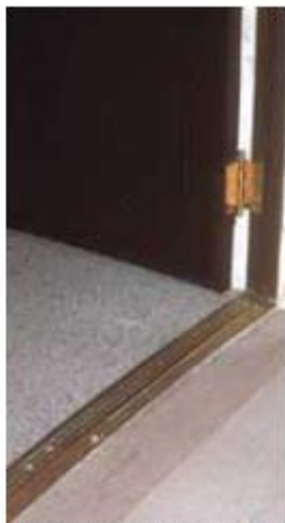
Historic threshold made accessible with 1/2" wood bevel.
