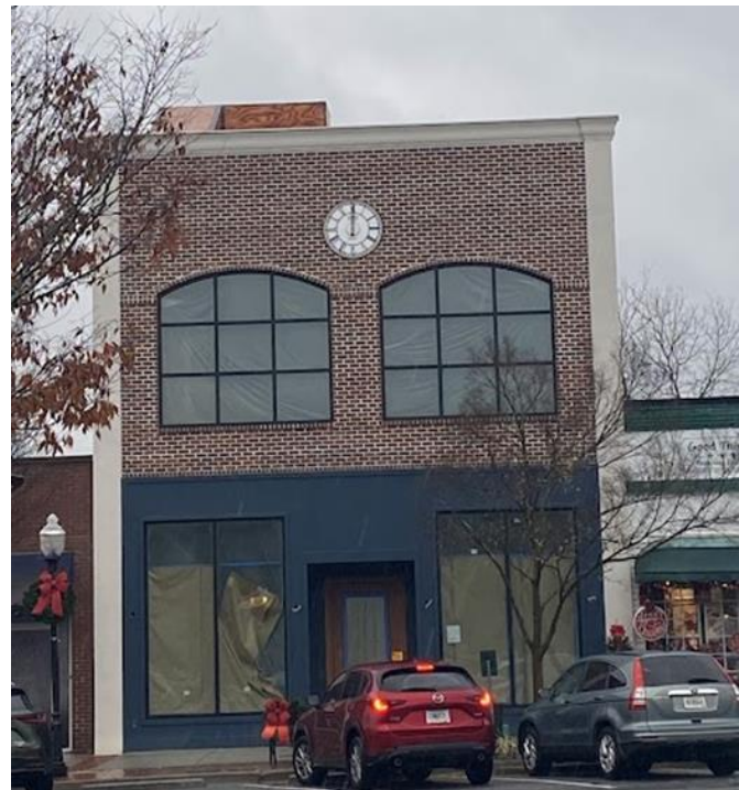
Existing Conditions – Photo Taken By Staff
