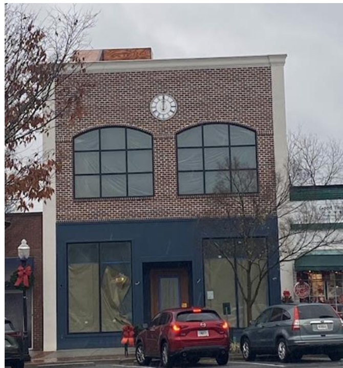
Existing Conditions – Photo Taken By Staff
