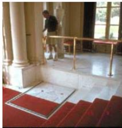
Compatible lift for historic foyer using "like" materials.
