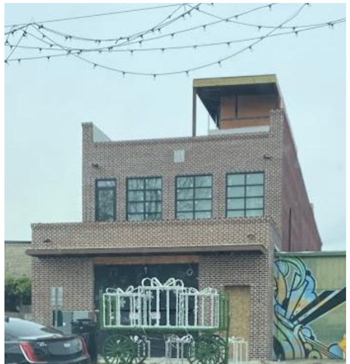
Existing Conditions – Photo Taken by Staff
