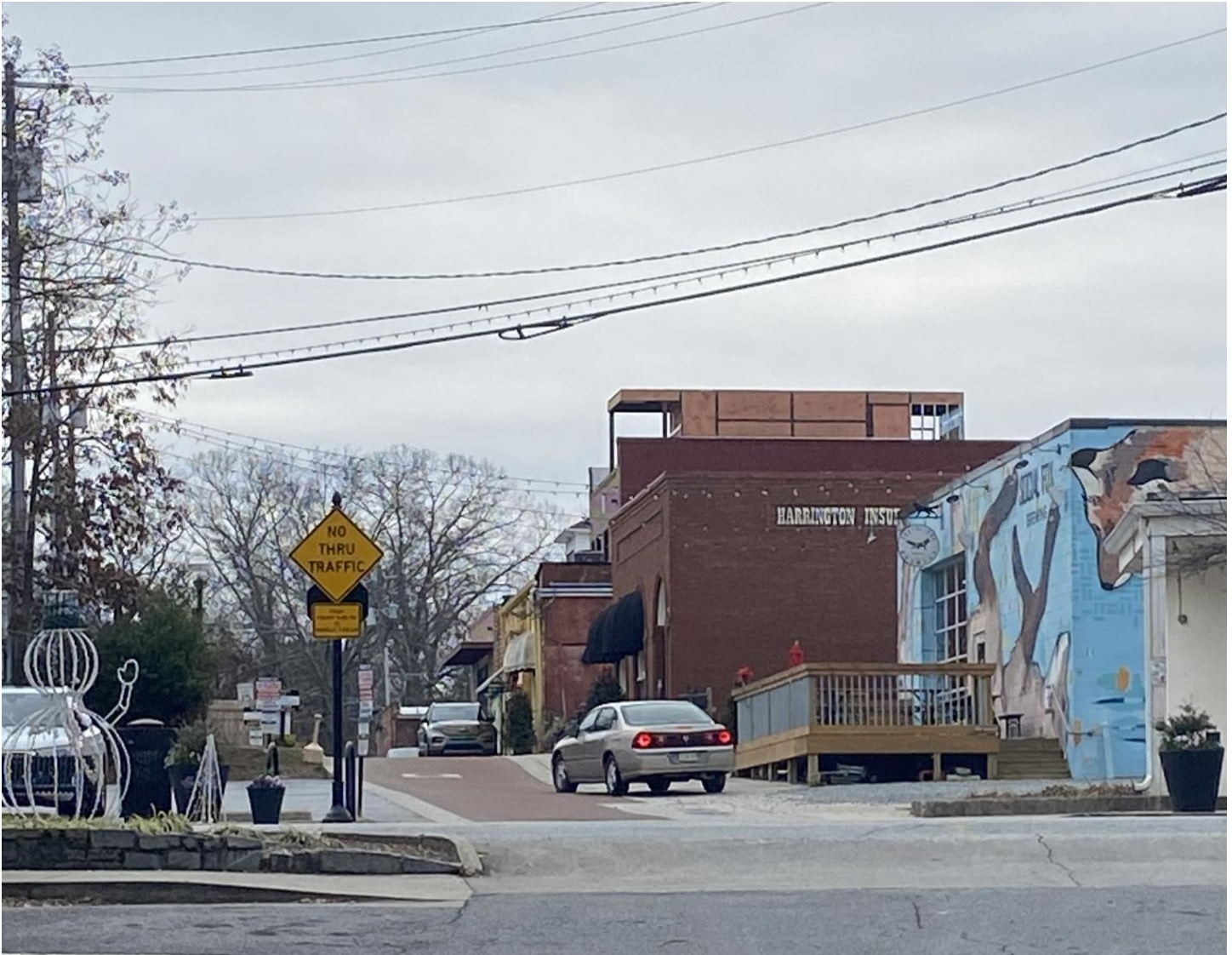
Existing Conditions – Photo Taken by Staff
