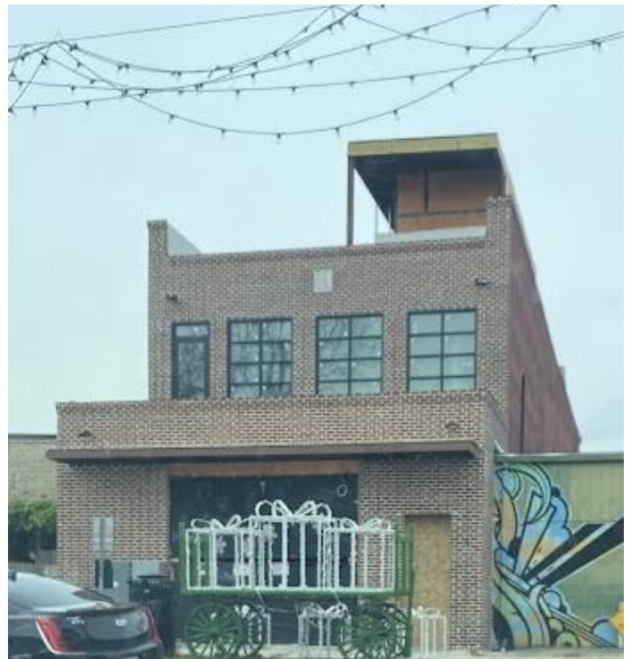
Existing Conditions – Photo Taken by Staff
