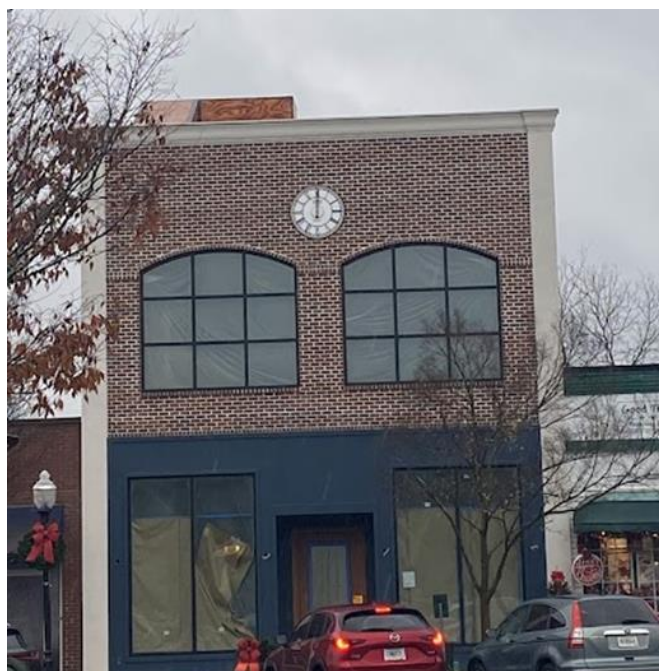
Existing Conditions – Photo Taken By Staff
