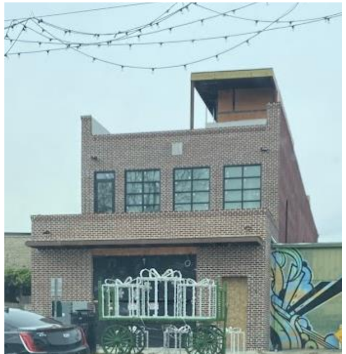
Existing Conditions – Photo Taken by Staff
