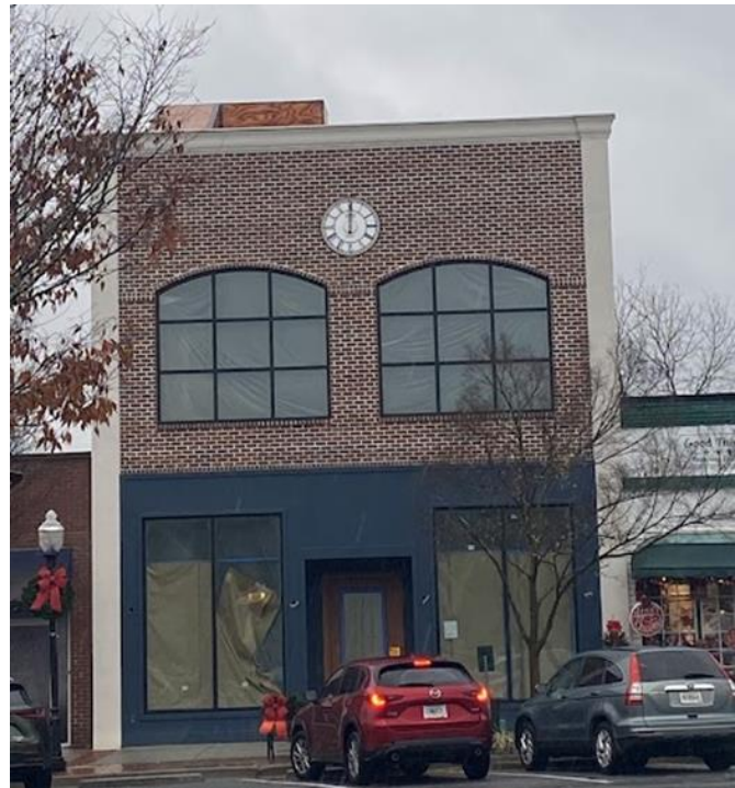
Existing Conditions – Photo Taken By Staff
