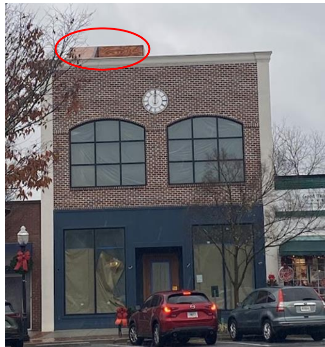
Existing Conditions – Photo Taken By Staff
