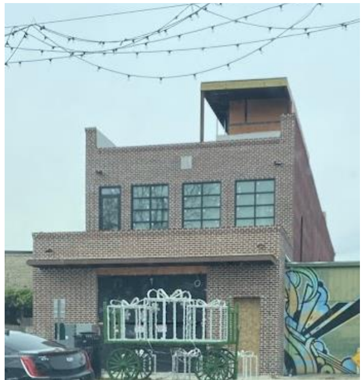
Existing Conditions – Photo Taken by Staff
