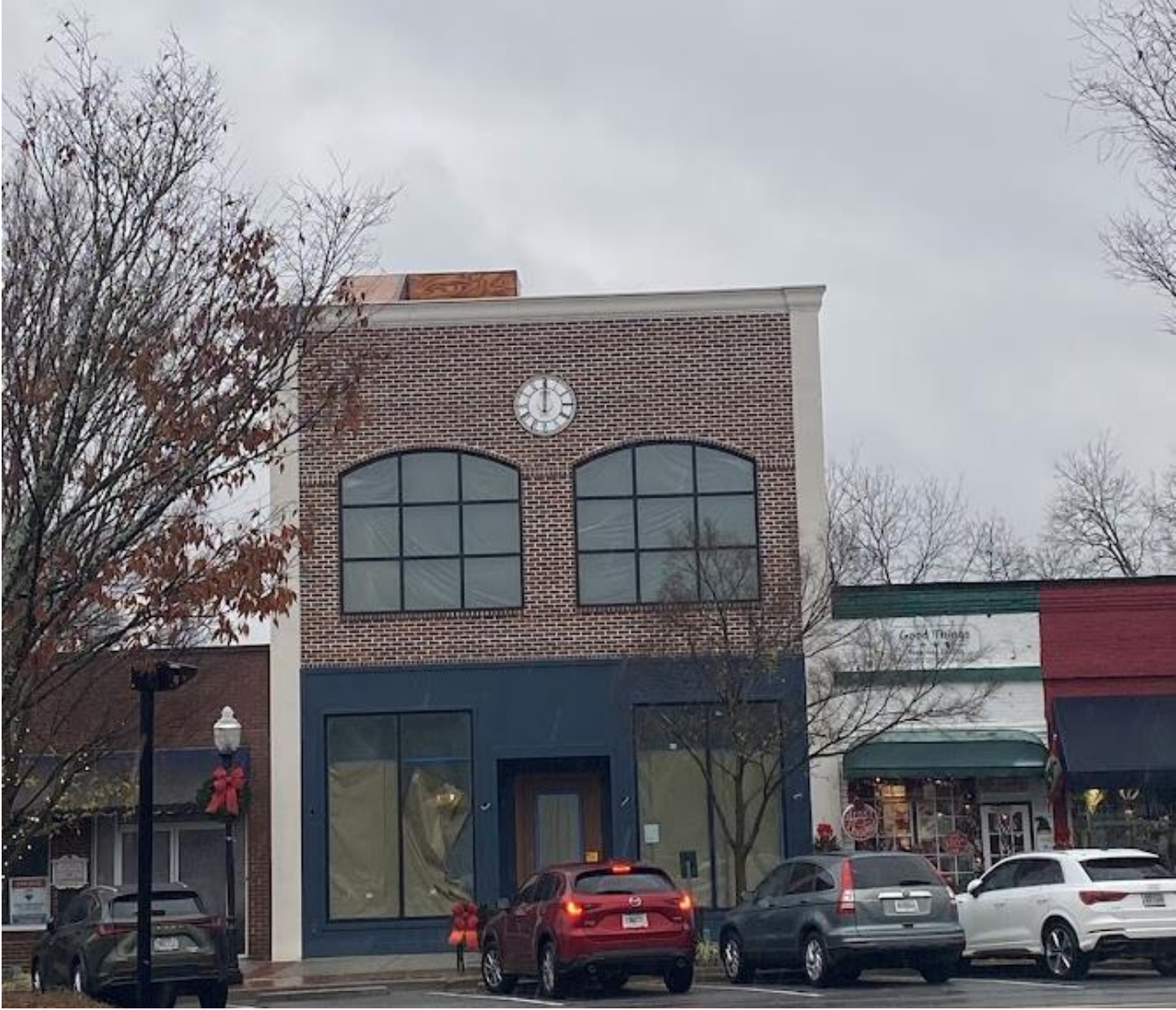
Existing Conditions – Photo Taken By Staff
