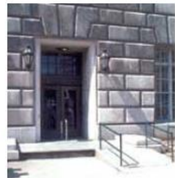
Entrance made accessible by adding inconspicuous ramp.
