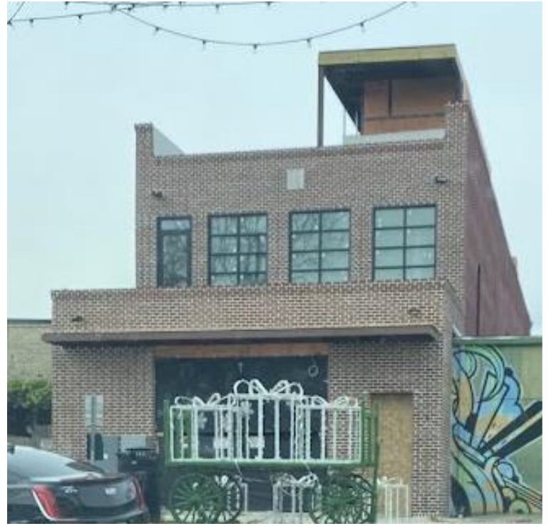
Existing Conditions – Photo Taken By Staff
