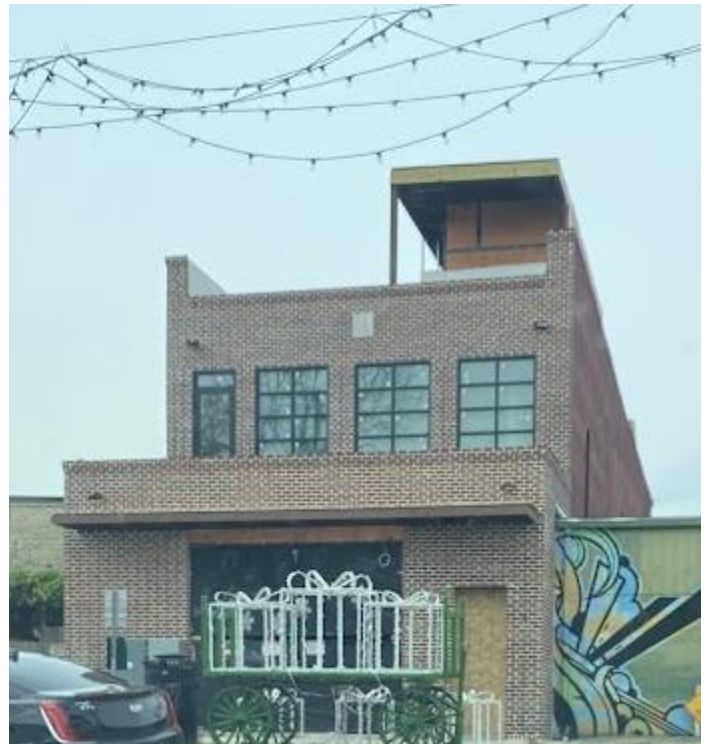
Existing Conditions – Photo Taken by Staff
