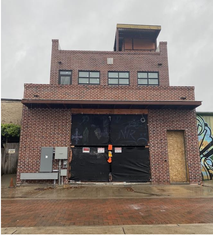
Existing Conditions – Photo Taken By Staff
