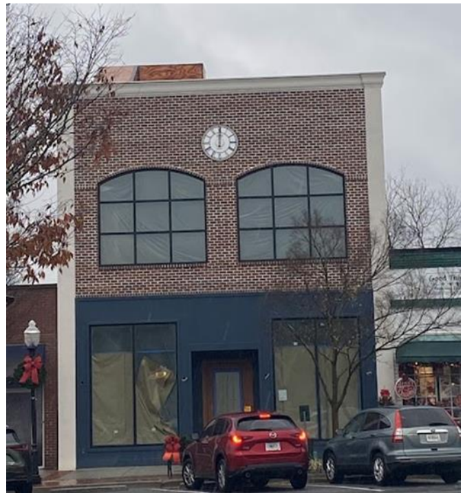
Existing Conditions – Photo Taken By Staff
