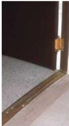
Historic threshold made accessible with 1/2" wood bevel.
