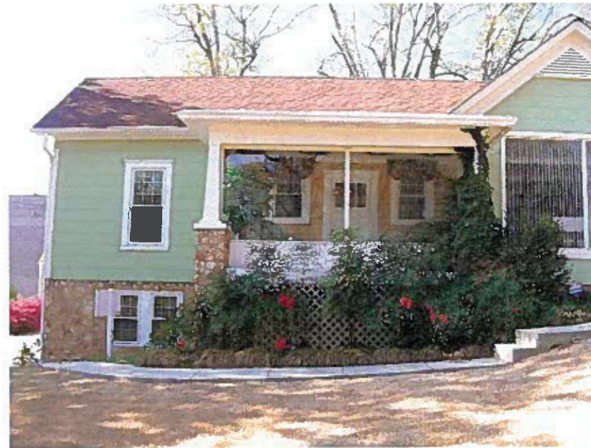
Photo 4: 207002 Burper Construction & Design Center
