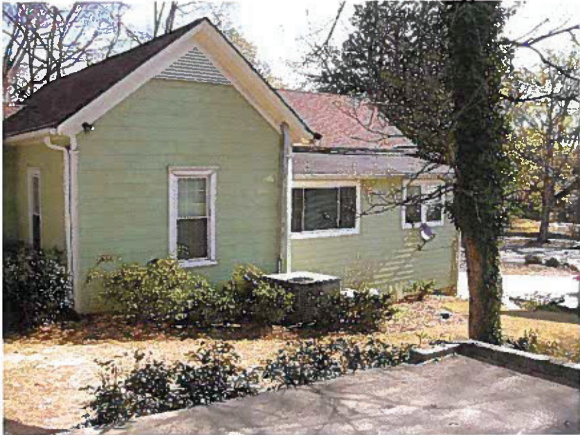
Photo 9: 207002 Burper Construction & Design Center
