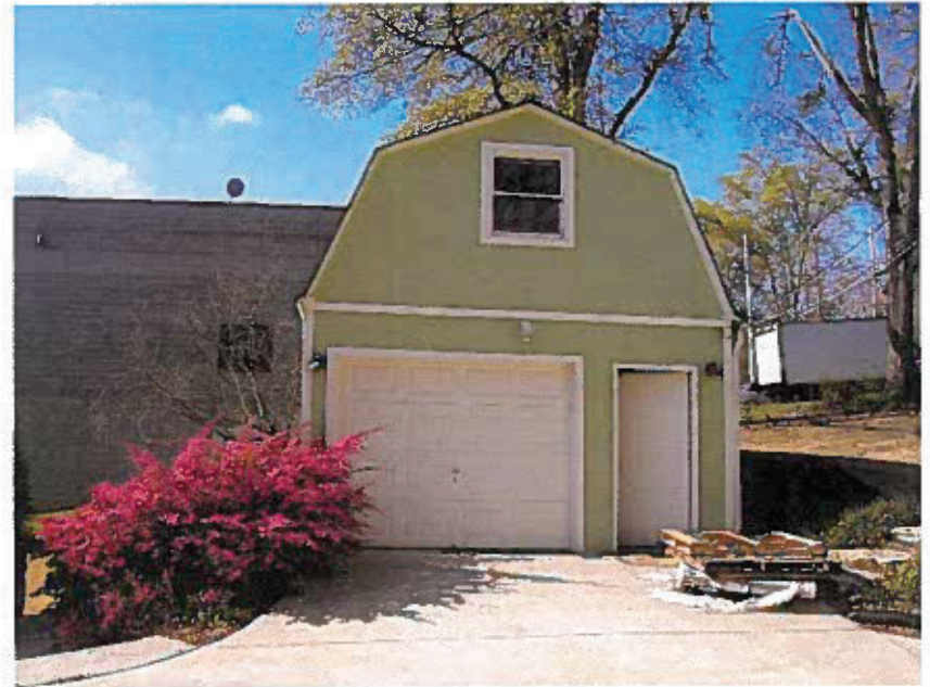
Photo 8: 207002 Burper Construction & Design Center
