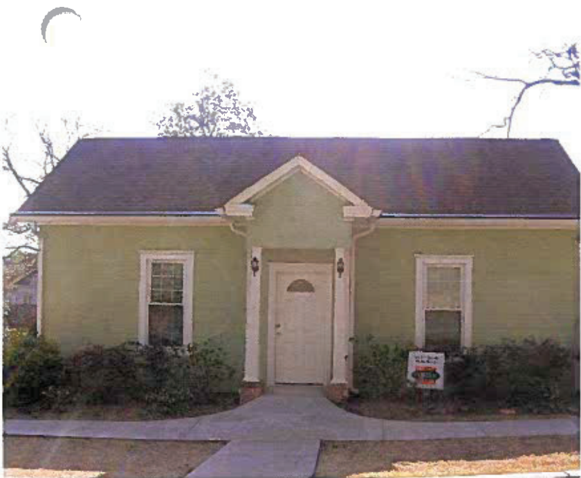
Photo 1: 207002 Burper Construction & Design Center
