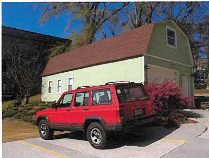
Photo 7: 207002 Burper Construction & Design Center
