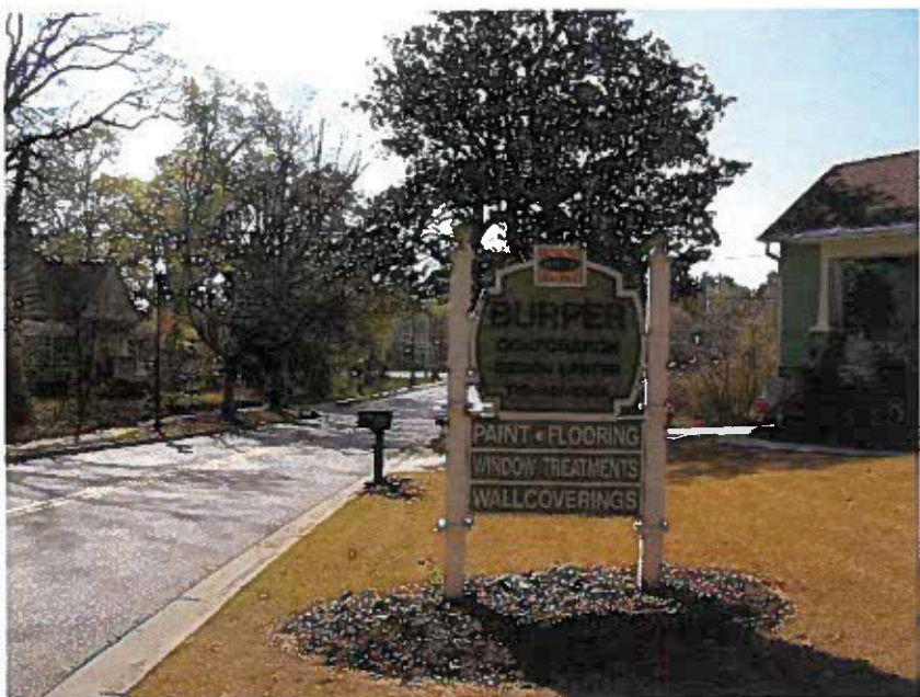
Photo 3: 207002 Burper Construction & Design Center
