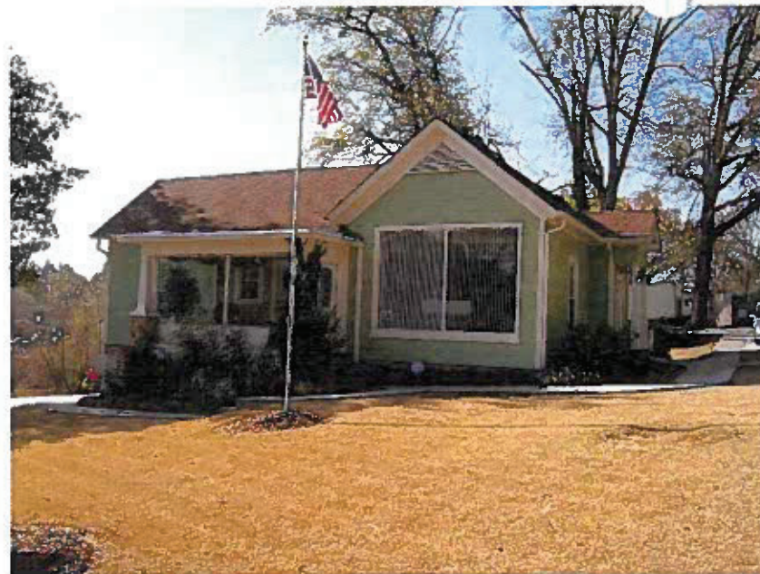
Photo 2: 207002 Burper Construction & Design Center
