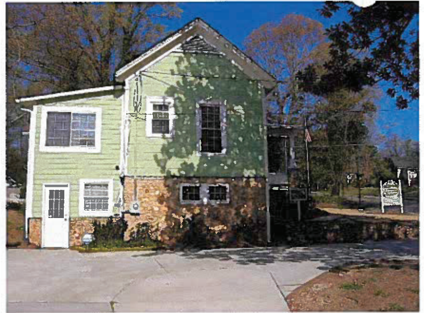
Photo 6: 207002 Burper Construction & Design Center
