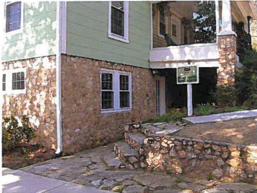
Photo 5: 207002 Burper Construction & Design Center
