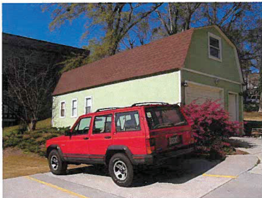
Photo 7: 207002 Burper Construction & Design Center
