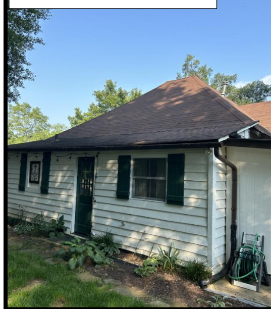
Existing Conditions (Rear)
