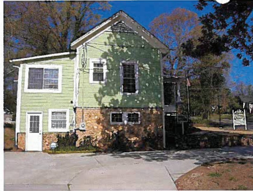
Photo 6: 207002 Burper Construction & Design Center
