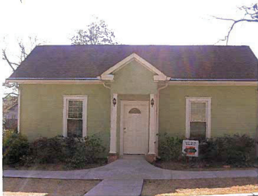
Photo 1: 207002 Burper Construction & Design Center
