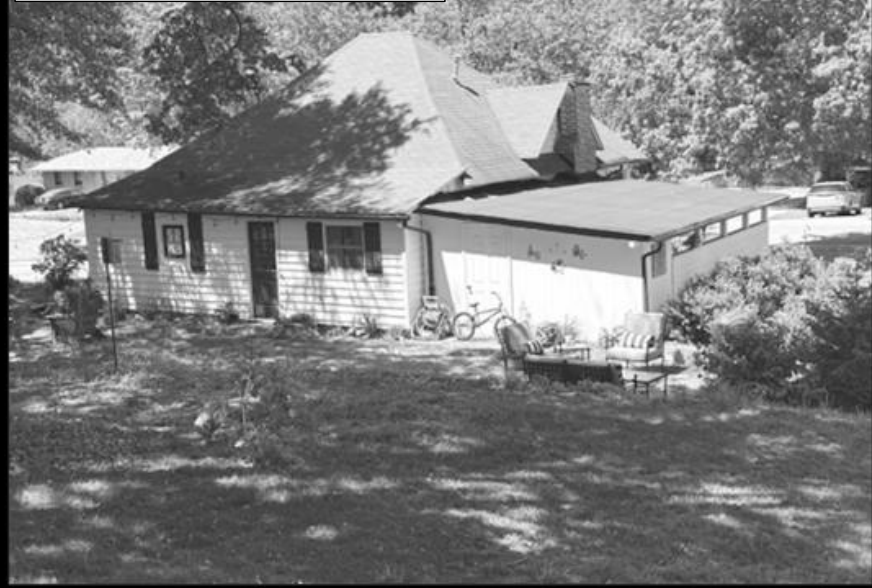
Existing Conditions (Rear)
