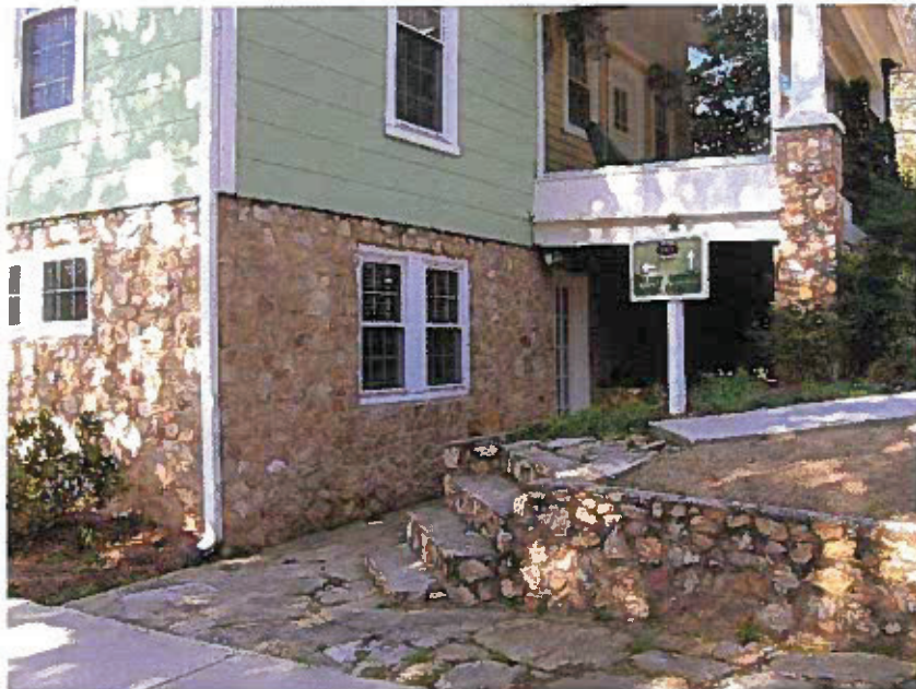
Photo 5: 207002 Burper Construction & Design Center
