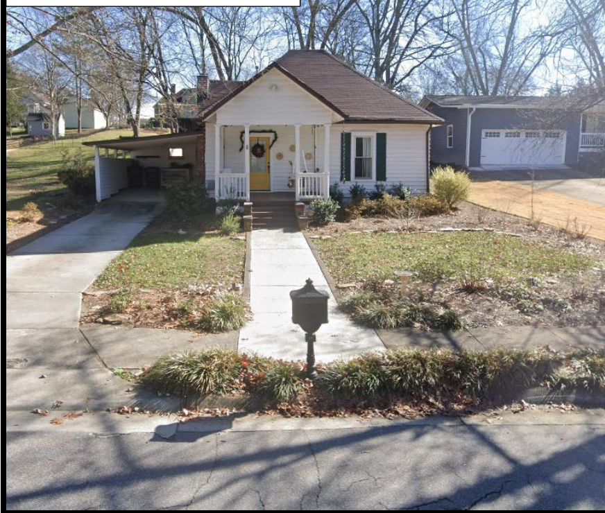
Existing Conditions (Front)
