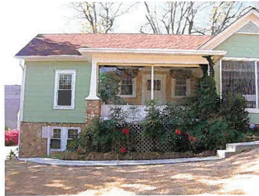
Photo 4: 207002 Burper Construction & Design Center
