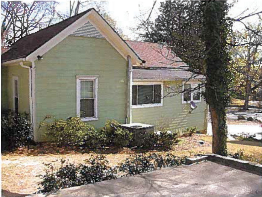
Photo 9: 207002 Burper Construction & Design Center
