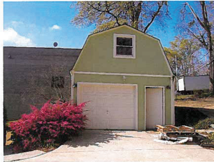
Photo 8: 207002 Burper Construction & Design Center
